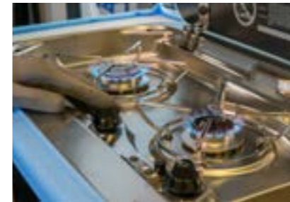
Test on operation of the gas pipes.
